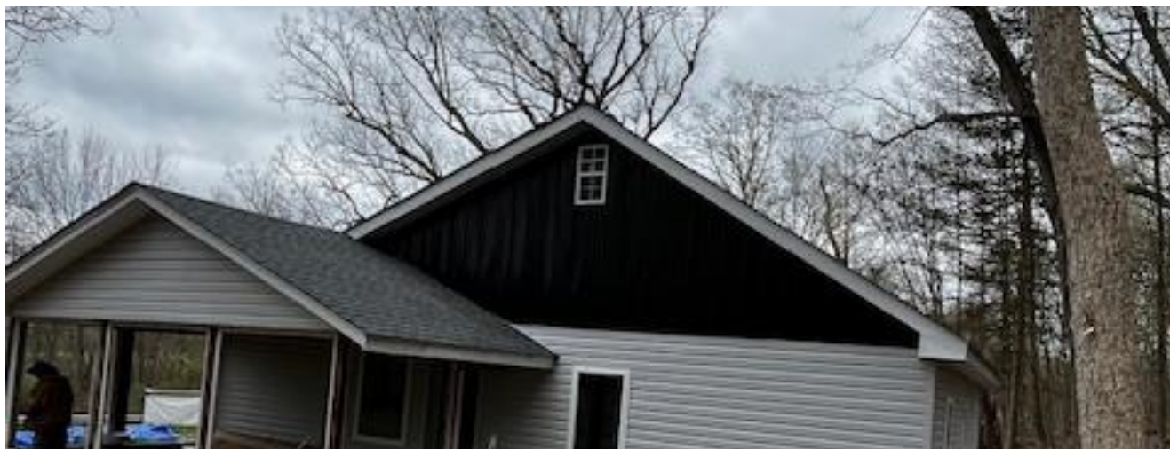
Another angle of 392 Rt. 565 — new siding, new windows, and a screened porch bring this Wantage home to life.
