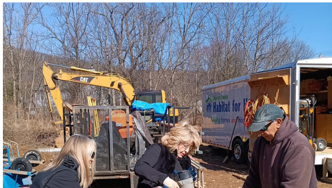
Volunteers on the Visions FCU team framing lumber, with the Habitat trailer close at hand.
