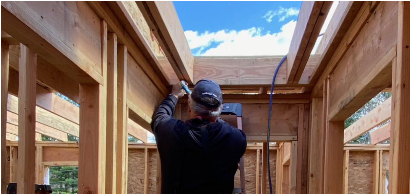
Volunteers working together on wall framing at 41 Mine Hill Road — the kind of teamwork that turns a foundation into a family's future.
