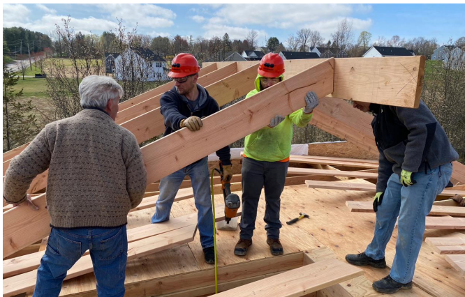
DSM Firmenich volunteers raised the ridge beam on April 9 — safety helmets on, spirits high.
