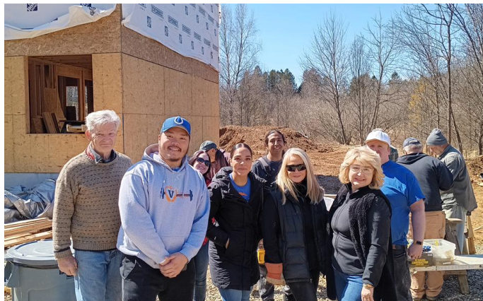
The Visions FCU team brought energy and commitment to the Mine Hill build on March 24.
