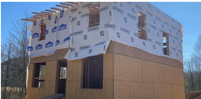
Mid-build: rafters reaching skyward as the home takes shape.
