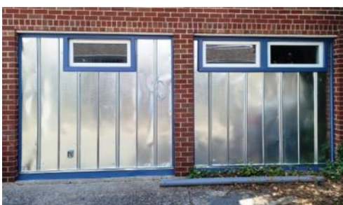
New installation at Community Center
